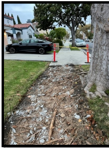
Sidewalk Panel Replacement with Root Pruning
